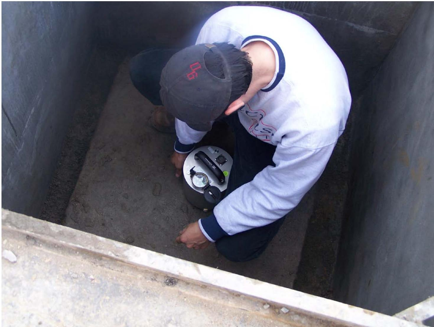
Installation of Seismometer at Sirala Station
